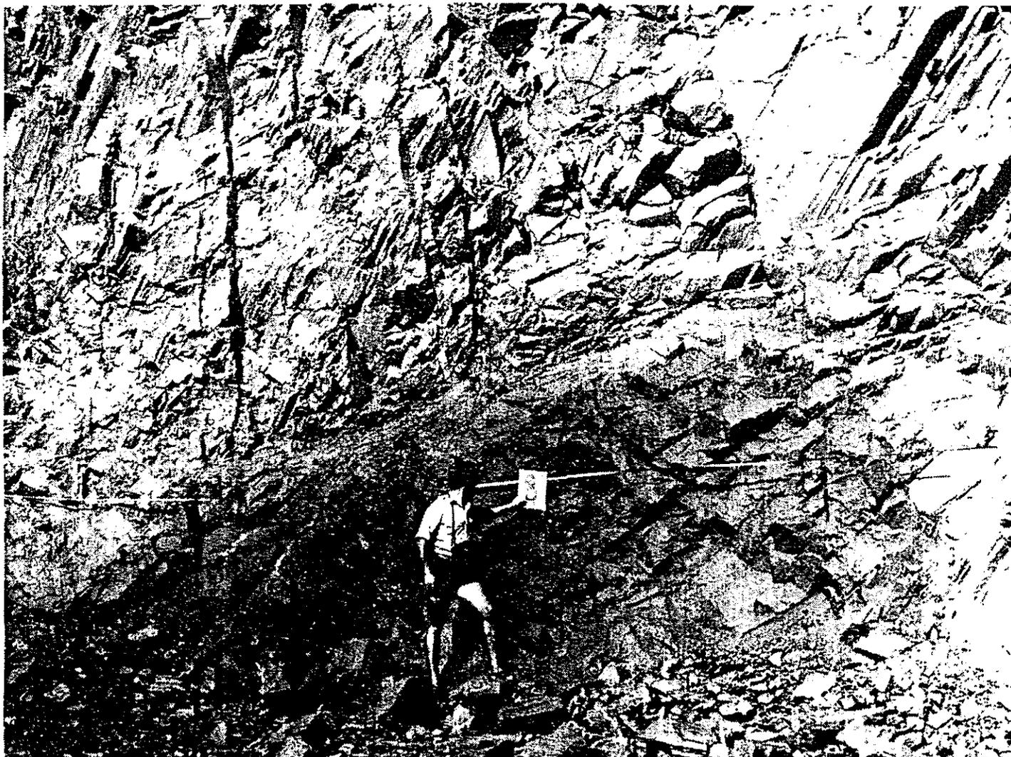
Figure 13. Appearance of Fractures in the Pit Face.
